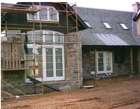
House near Perth by SIPit(Scotland) Ltd
