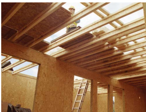
Engineered floor joists in SIP house
