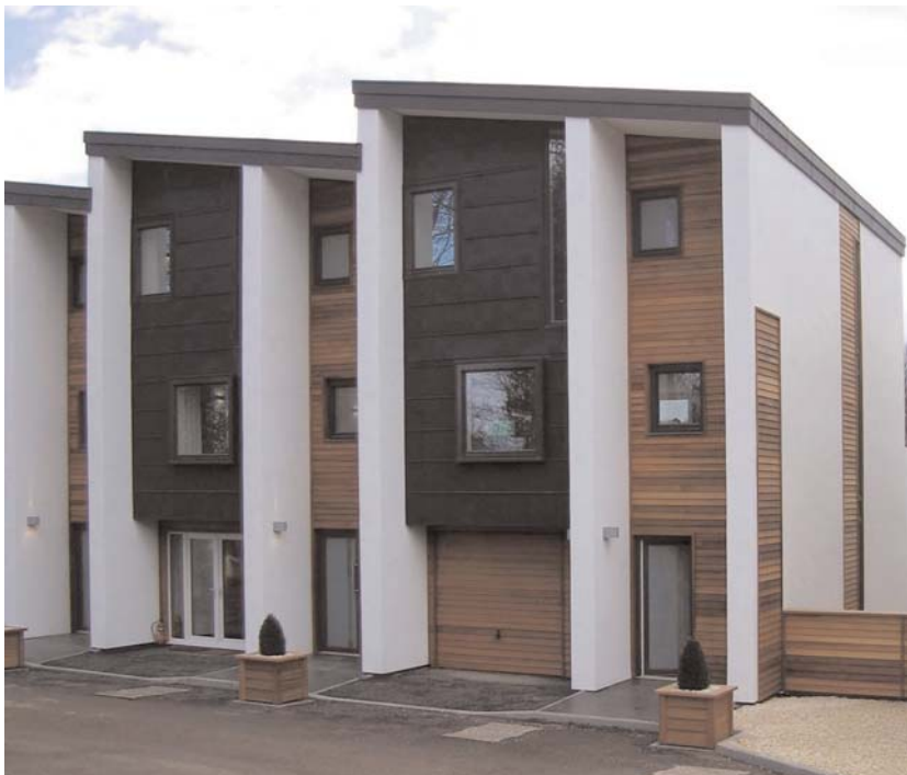
Modernist town houses in Newcastle by SIPit (Scotland) Ltd
