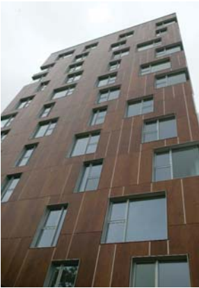
Tall building clad in SIPs supplied by SIPBuild
