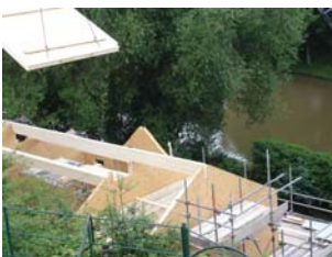
Erecting panels by crane above and by hand below
