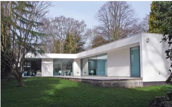
Modernist house supplied by SIPBuild
