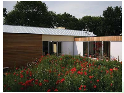
Modernist house supplied by SIPBuild
