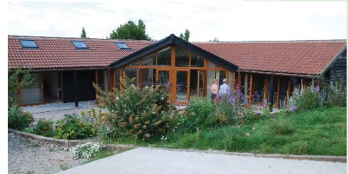
Modern bungalow designed for disabled occupant supplied by Edward Halford Ltd
