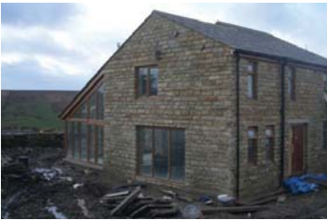
SIP buildings by SIPBuild
