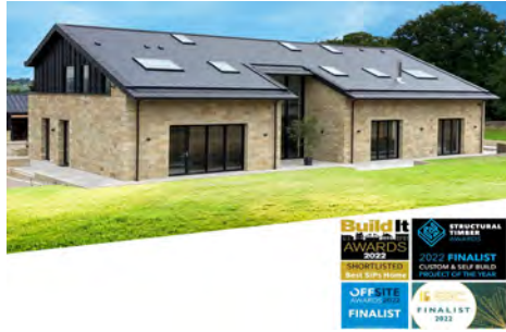
Hampsthwaite | SIP Self Build Project
